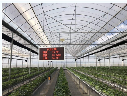
Typical greenhouse installation
